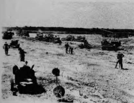
PREPARATION OF SUB-GRADE
