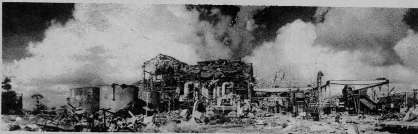
DEMOLISHED JAP SUGAR MILL
